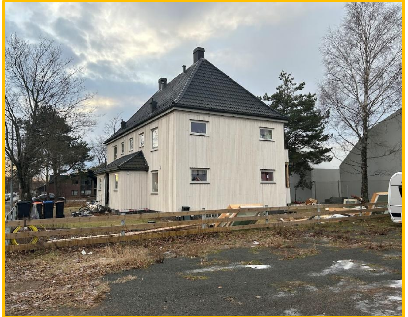
Skiringsalsgata 25. Under rehabilitering, ferdig Q1 2024
